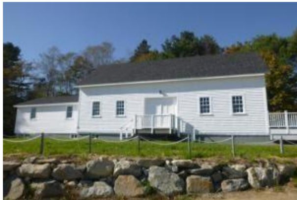
Relocated museum in place and secured
