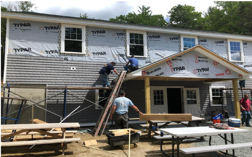
Independent Order of Odd Fellows New Lodge - at 620 Bagaduce Road
