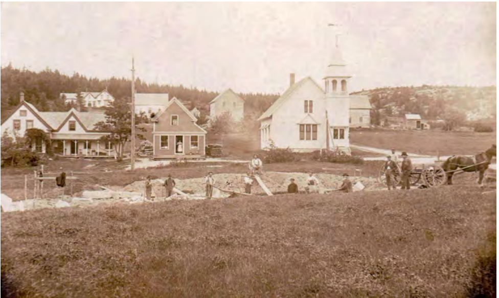
Laying a foundation in Buck's Harbor. Mell Condon's Store across the road with Clara standing in doorway
